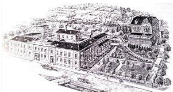
The F.X. Hüller & Co factory and house around 1920, source: Hüller & Co catalog
