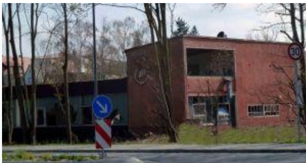
The Emo factory in Diespeck, built in 1954, extended in 1956. In 2017 it was removed to build a home for the elderly
