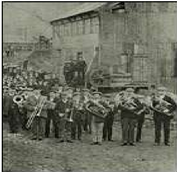
(Nenthead Band 1902 – At Rampgill Mill)
